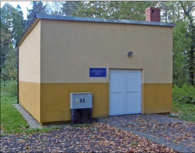
Hydrofornia w Jezierzycach (SHR) po remoncie.
